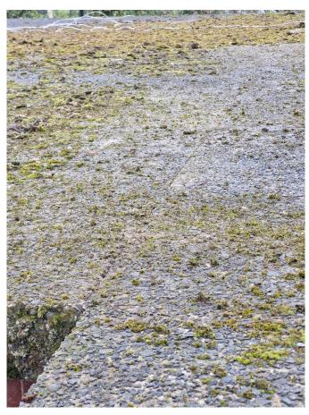
Viewed from the inside the location of the leaks was readily apparent and has created some damage to the ceiling. Viewed from the outside the joint is visible, but also visible is the moss growth which is also retaining some of the water on the roof.
